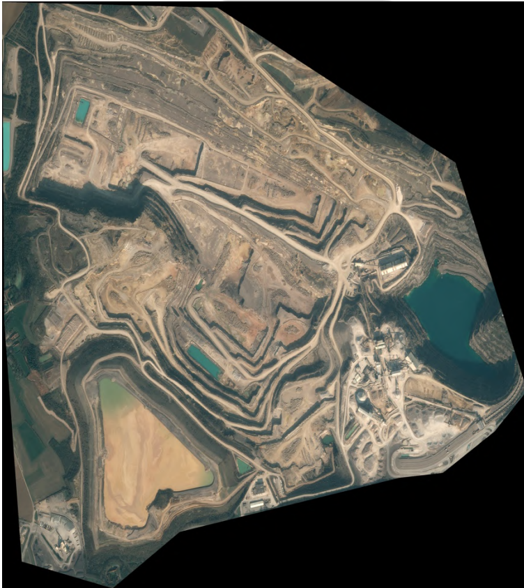
Figure 7 : Photo of the quarry on 20 march 2022
