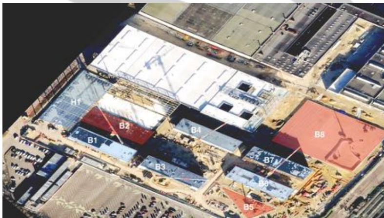
Figure 13 : Annotated construction site
